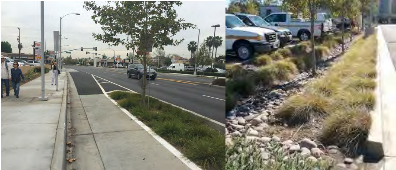
Left - Protected bikeway with integrated bioswale, Temple City, CA, Right - Bioswales adjacent to parking lot in San Diego, CA
