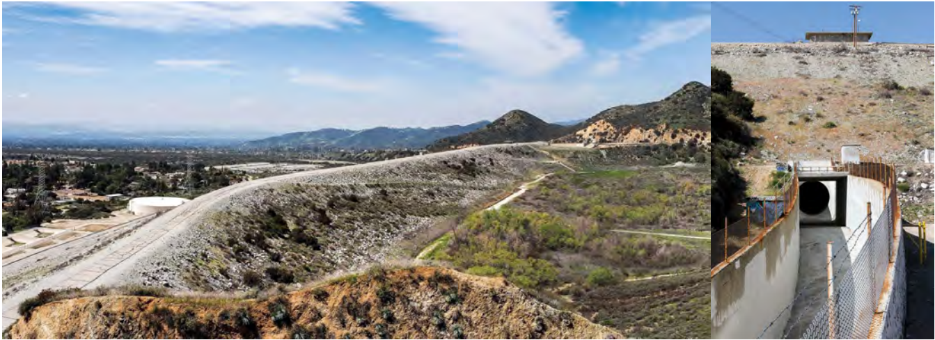
(Left) San Antonio Dam and filling basin, (Right) San Antonio Creek emerges from Dam (image source: Spencer Croce)
